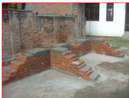
Load Bearing Wall
